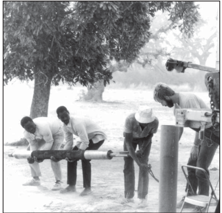
Ray Boyle hydrofracturing with a Fracker™ in Africa
